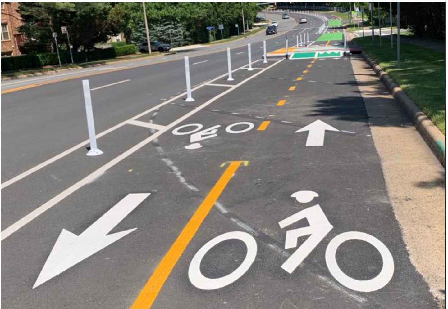
New Bike lanes at Vienna Metro, Virginia Center Drive
