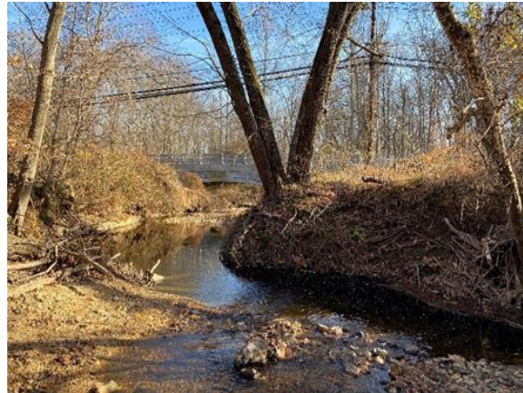
Overhead electric lines and road bridge at end of stream segment 0030-008.
