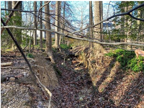
Widening outfall channel.
