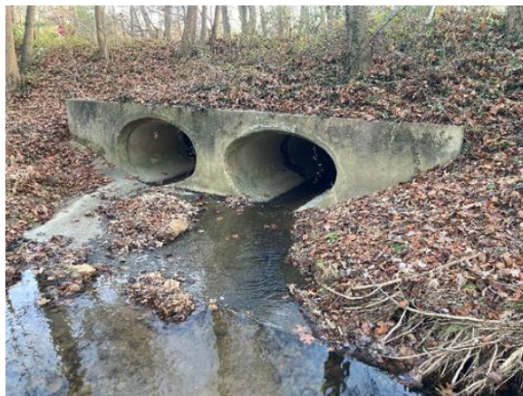
Double culvert at downstream project limits.
