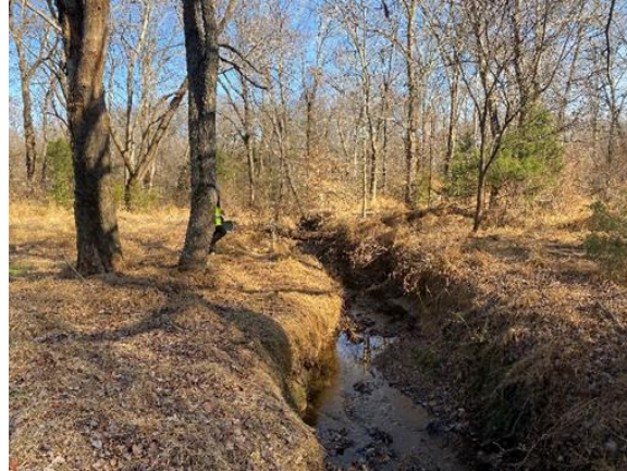
Widening channel with actively eroding banks and lack of trees.
