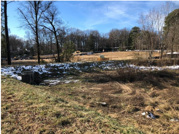
Nearby construction, restriction for expansion or lowering embankment on southern side of pond.
