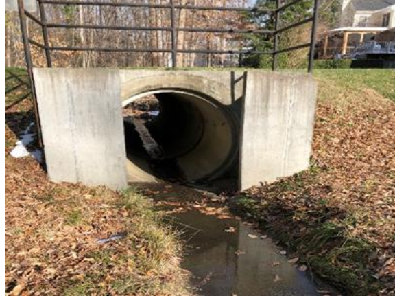
Flow control structure in front of outlet culvert.
