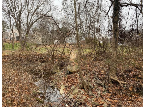
Paved outfall ditch discharging into stream.
