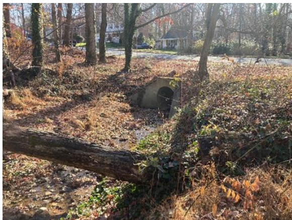
Stream segment entering the downstream culvert that passes under Braeburn Drive.
