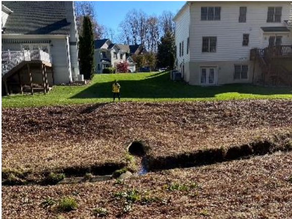
Access in between residential properties.
