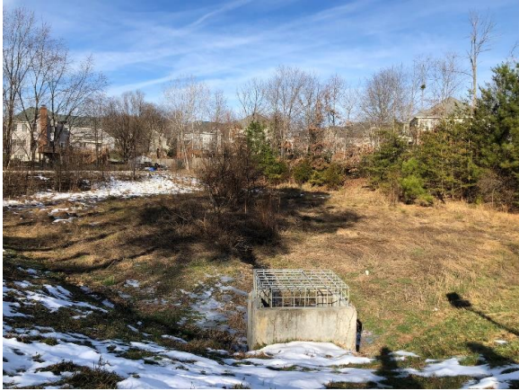
Channel entering riser, trees on pond embankment and vegetation in basin.
