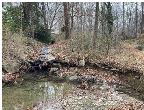
Concrete outfall channel discharging into widening natural channel.
