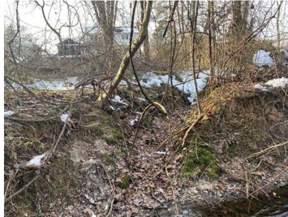
Widening outfall channel.
