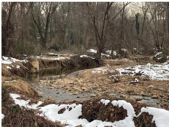
Entrenched, widening stream channel impeding on infrastructure; large supply of streambed material.
