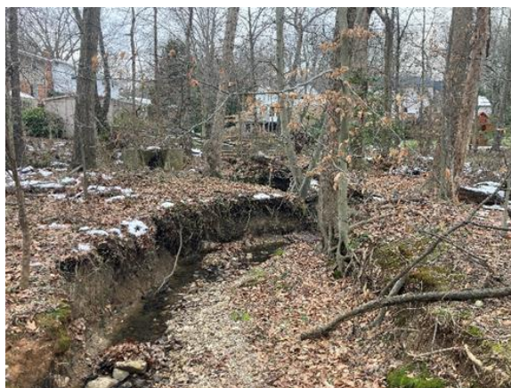
Widening outfall channel.
