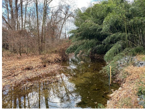
Widening channel with large invasive plant species along left bank.
