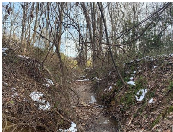
Incised, widening outfall channel.
