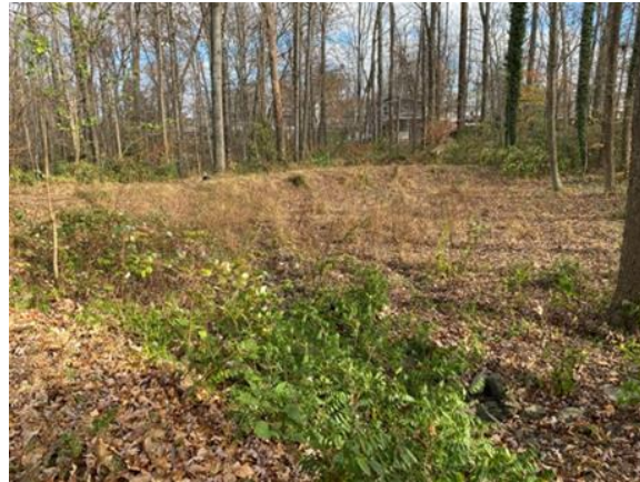
Existing peak shaver dry pond.
