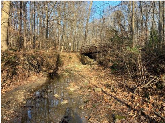
Incised and widening channel.
