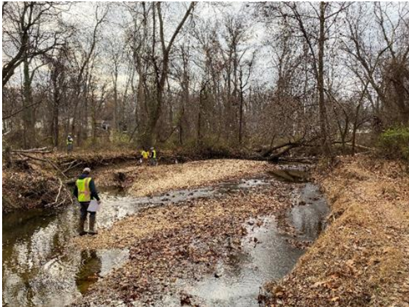
Entrenched, widening channel with multiple flow paths due to mobile substrate; large streambed material deposit.
