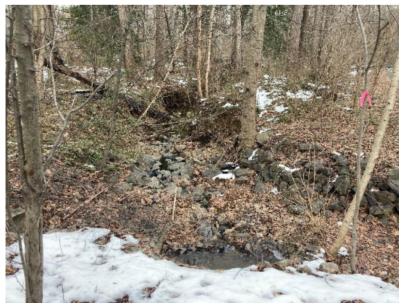
Trail culverts discharging into stream segment.
