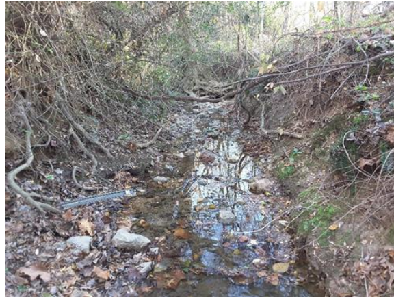
Example of a widening outfall channel.
