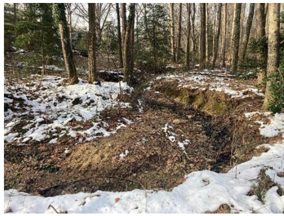
Eroded tributary with existing bench.
