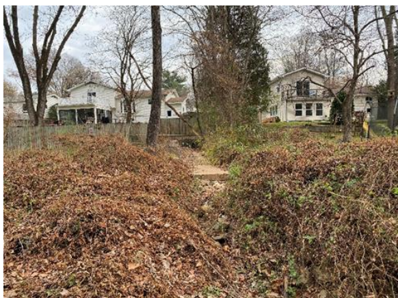
Impervious outfall channel with invasive plant species as dominant floodplain vegetation.
