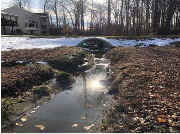
Culvert and side channel directing flow to concrete ditch.
