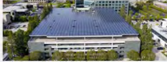
Parking Structure Photovoltaic Shade Structures
