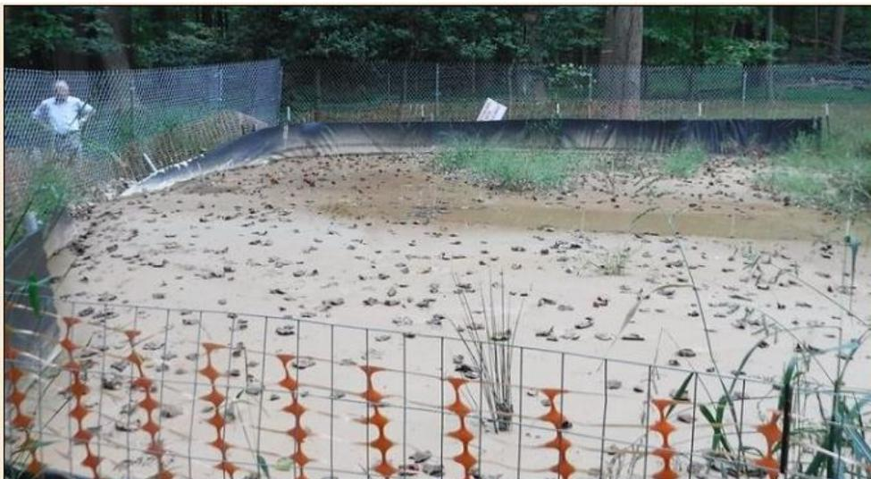
*Before citizen report - Neglected silt fence filled beyond capacity, overflowing sediment into stream*
