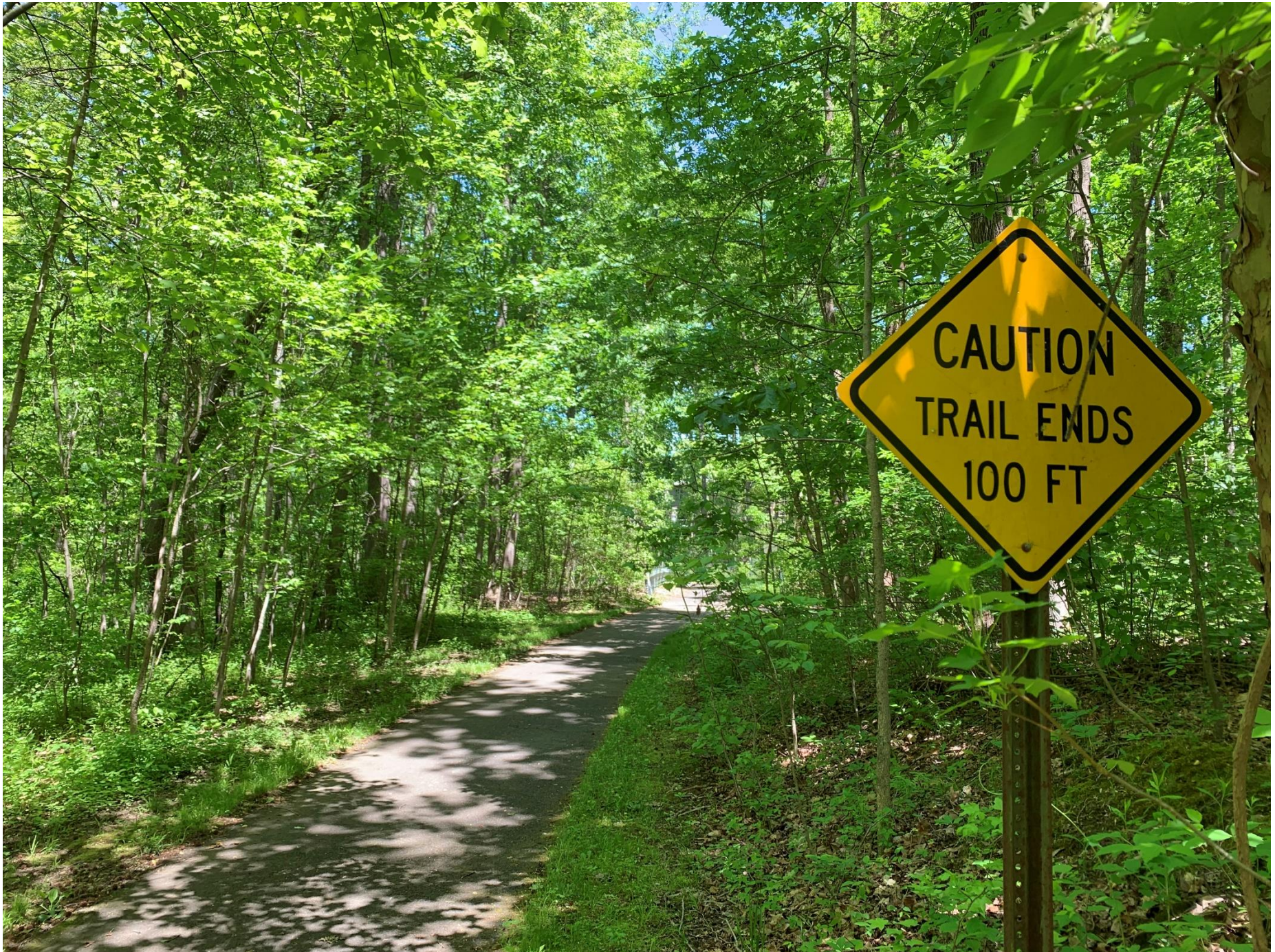
Unfortunate recent northern extension of existing Island Creek Park paved trail
