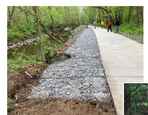
**Left:** Originally asphalt, this section of Fairfax County's Cross County Trail washed away and had to be replaced with more durable concrete (twice as expensive as asphalt). New gabion reinforcements have now been added to prevent it eroding into Accotink Creek, adding more maintenance issues.
