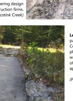
**Left:** In under 3 years, asphalt paving of this section of Fairfax County's Cross County Trail was physically displaced by flowing waters. (Also note the wide right of way cleared for this approximately 8' wide path)
